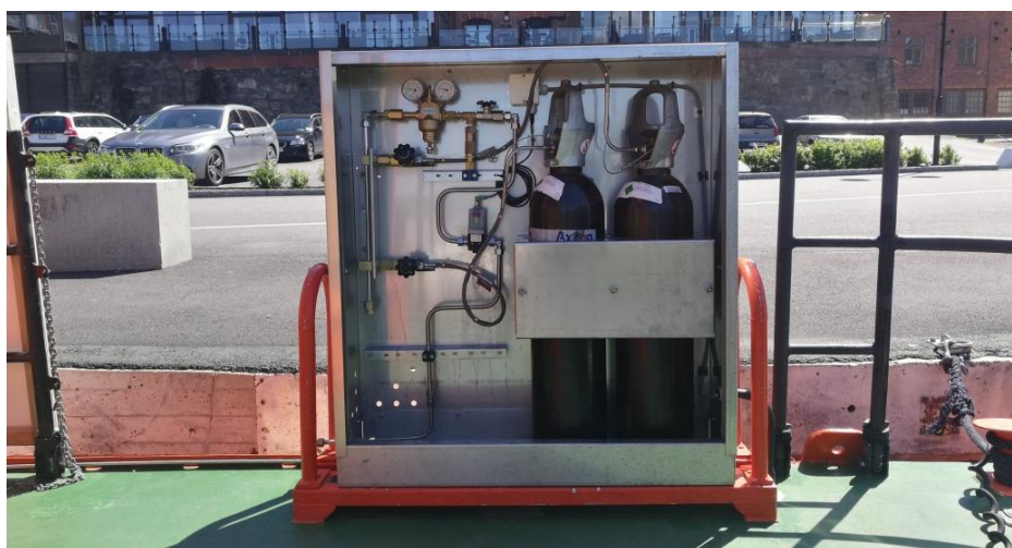
Figure 2-5: The nitrogen cabinet on deck. Two bottles are connected but one is in use.
