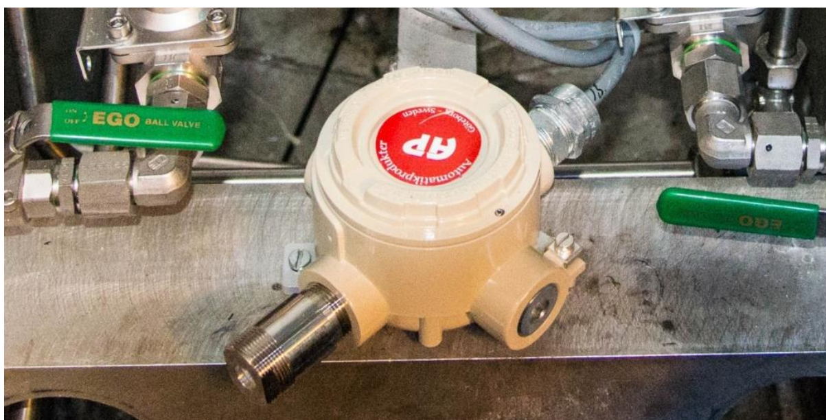
Figure 2-12: The gas detector in the methanol tank room. Also partly visible are the manual and solenoid master fuel valves for the methanol tanks.
